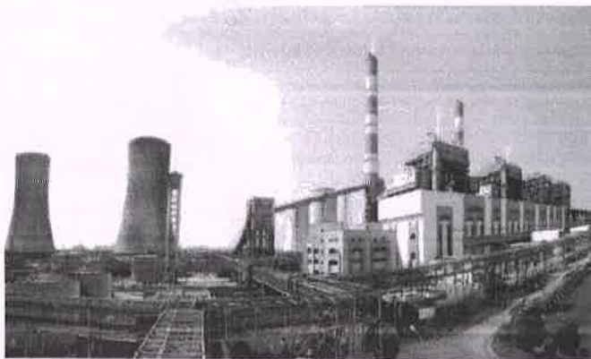
Coal based thermal power plant in India
